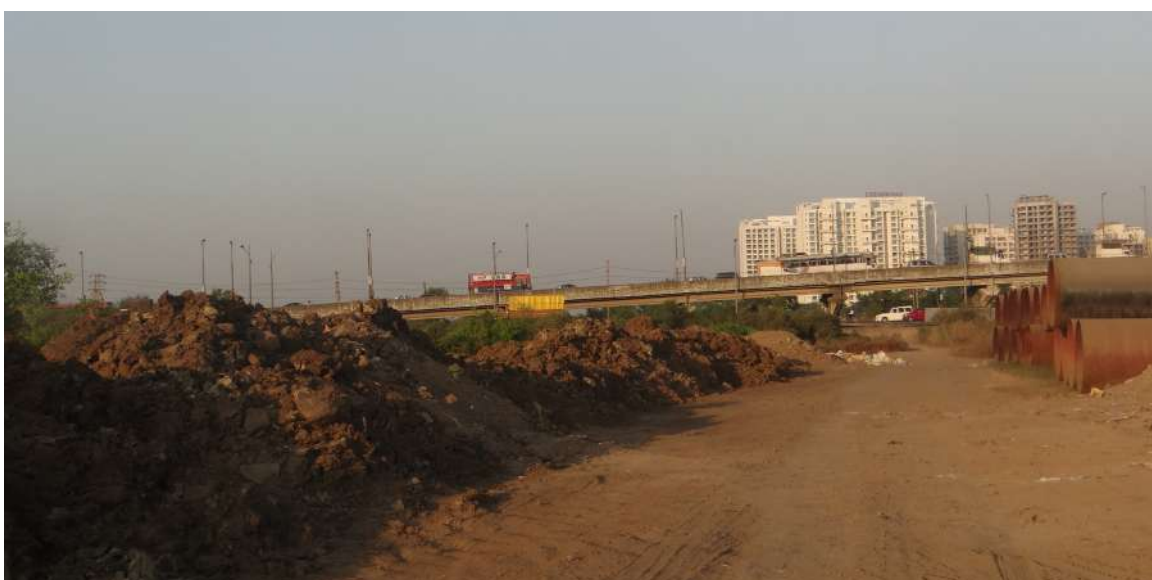
Laying of pipeline
