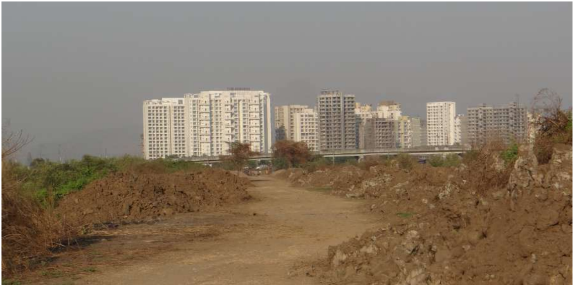
Construction of roads through salt pans and mangroves
