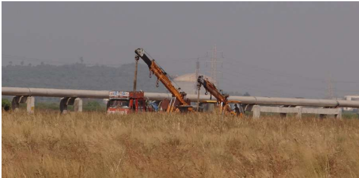
Area after landfilling opposite to Nava Sheva Police Station
