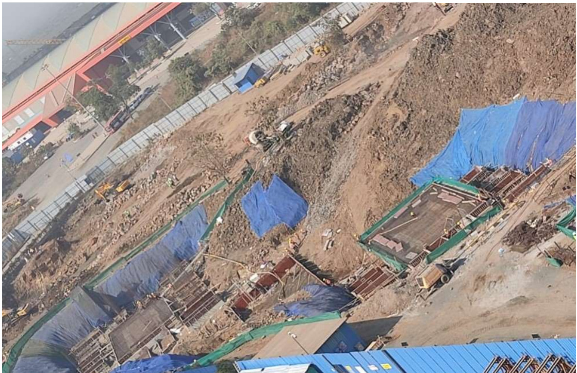
Figure 9: Excavation Activity On site
