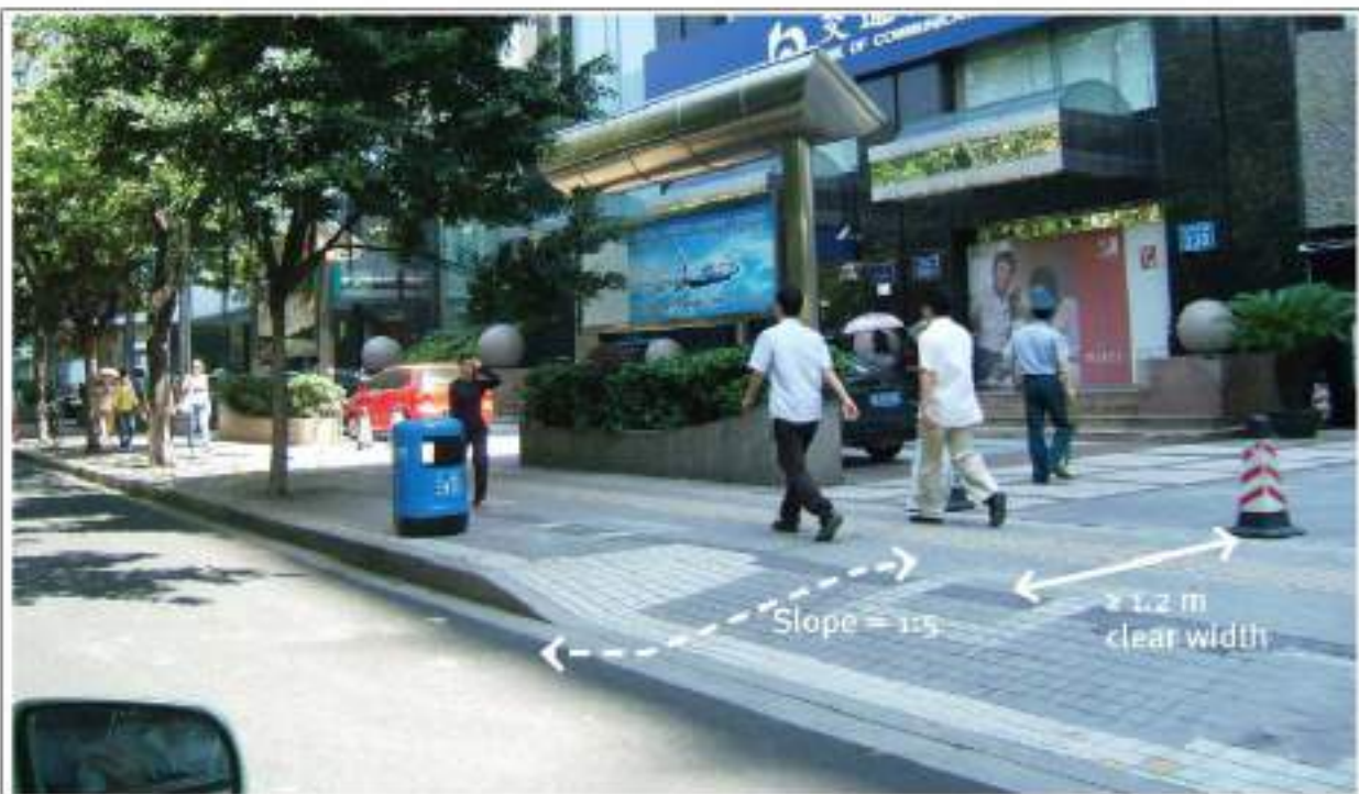
CONSTRUCTION OF FOOTPATHS AT PROPERTY ENTRANCES
