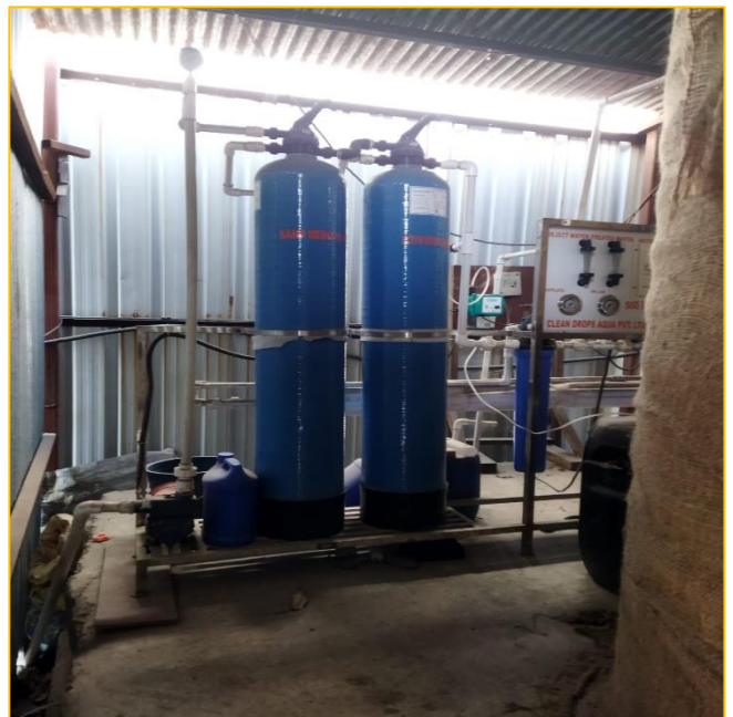
RO Plant installed at site for drinking water.
