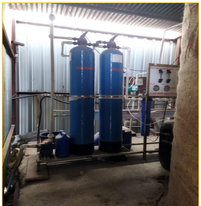
RO Plant installed at site for drinking water.
