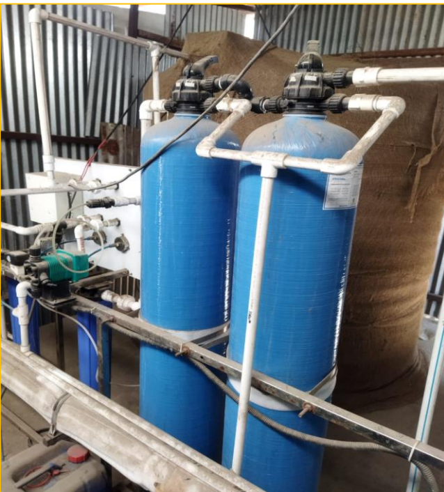
RO Plant installed at site for drinking water.
