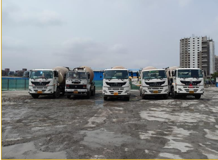
Annexure – 11: Vehicle parked only inside of project.
