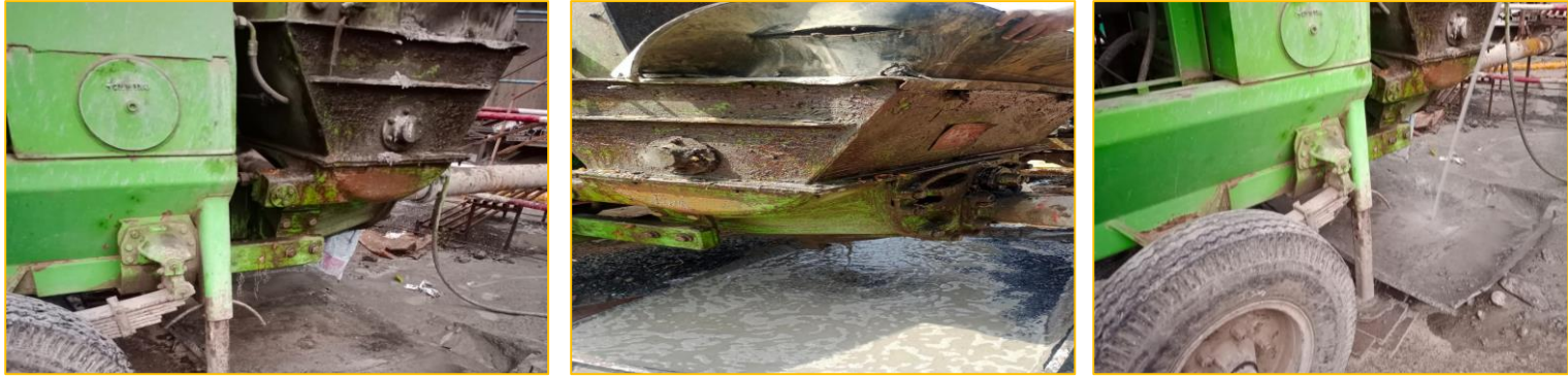
Deep Tray Provision is being followed at site for concrete pump wash to prevent soil contamination.
