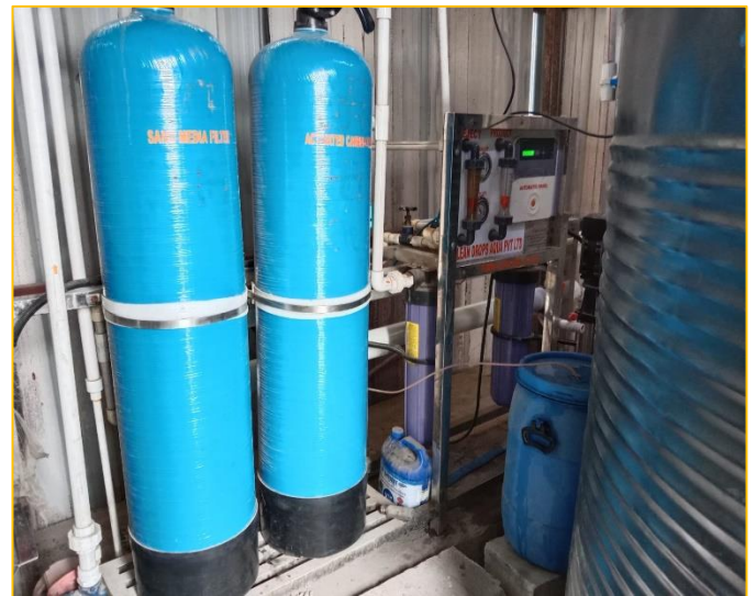
RO Plant installed at site for drinking water.
