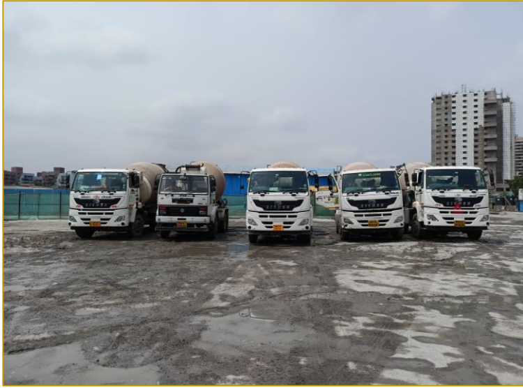
Annexure – 11: Vehicle parked only inside of project .
