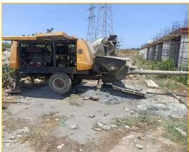
Deep Tray Provision is being followed at site for concrete pump wash to prevent soil contamination.
