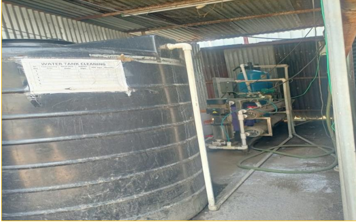
RO Plant installed in Workmen Camp for drinking water.
