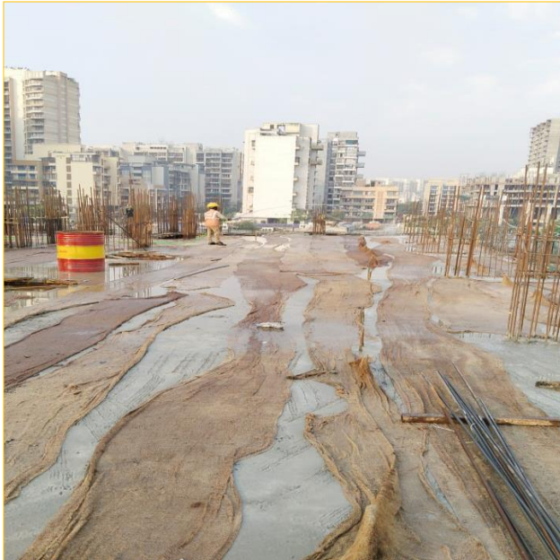
Annexure - 09: Hessian cloth used to curing during construction.
