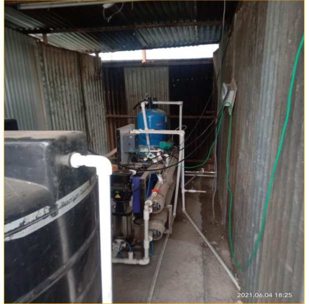
RO Plant installed in Workmen Camp for drinking water.
