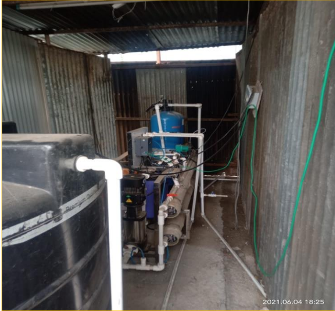
RO Plant installed in Workmen Camp for drinking water.
