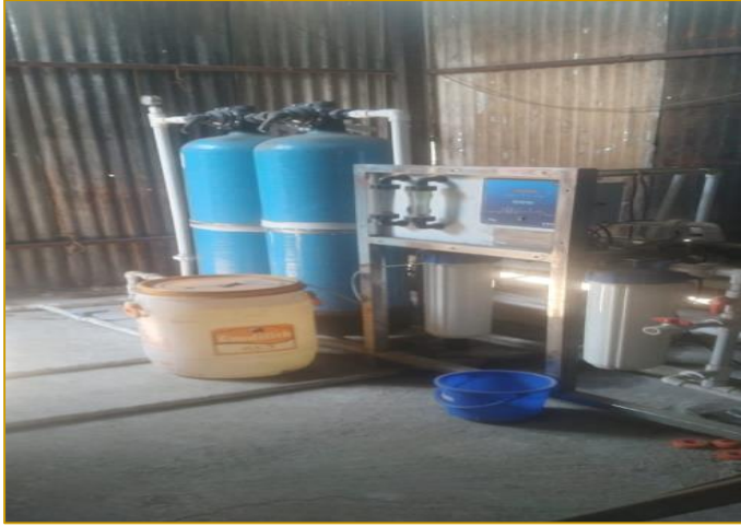
RO Plant installed at site and Workmen Camp for drinking water.
