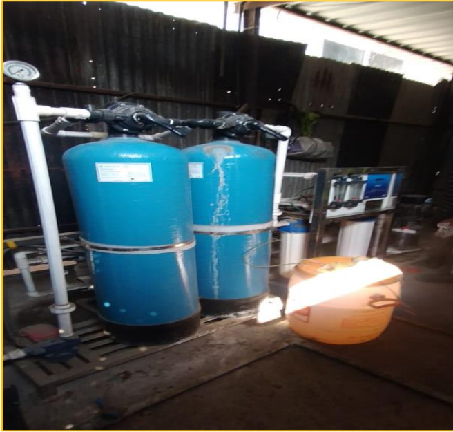
RO Plant installed at site and Workmen Camp for drinking water.
