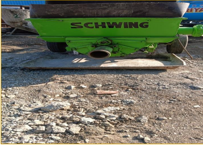
Deep Tray Being used at site for Concrete pump wash to avoid soil contamination.
