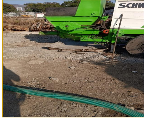
Deep Tray Being used at site for Concrete pump wash to avoid soil contamination.
