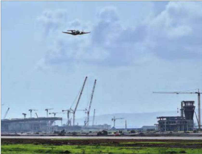
The Airports Authority of India on Monday started conducting flight calibration of the instrument landing system (ILS) at the under-construction Navi Mumbai International Airport. The ILS provides horizontal and vertical guidance to pilots while approaching the runway. The airport is expected to start the first phase of operations by March 2025. BACHCHAN KUMAR/ HT PHOTO
