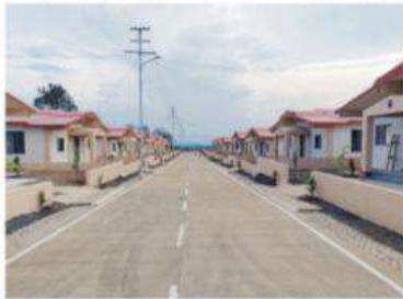
The newly constructed houses for the survivors
