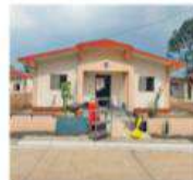
One of the survivors shifting his belongings into the new constructed houses
