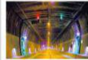
The Kharghar-Turbhe tunnel road will provide direct connectivity between Turbhe on north Navi Mumbai and Kharghar in south Navi Mumbai
